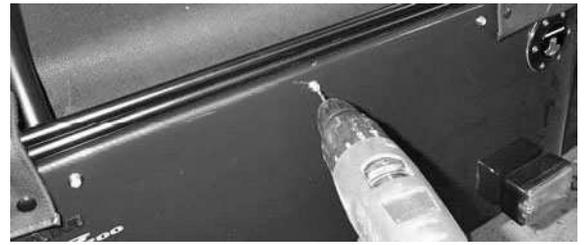
Fig 22 Drilling central popper on SV
